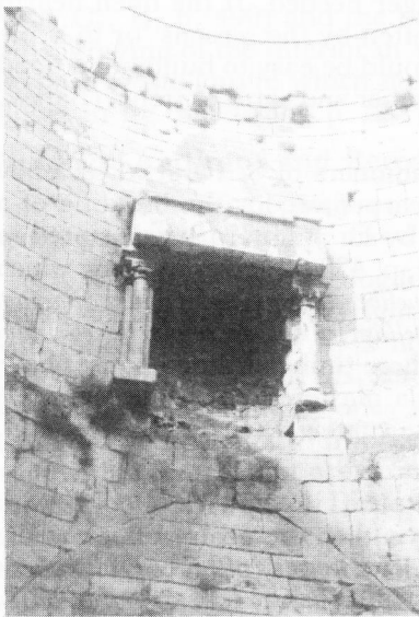
Fig. 7 A fireplace in the sophisticated keep of Conisborough Castle, Yorkshire, with a canopy and toggled lintel, c. 1190
